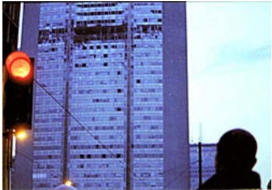
Fig. 2 - The Pirelli tower after the accident
